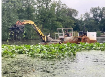
Dredging Project to clear outfalls in Camden City to improve functionality.
