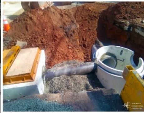
Installation of catch basins to control the flow of storm water as part of Ridgefield Park Village's long term control plan to address CSO's
