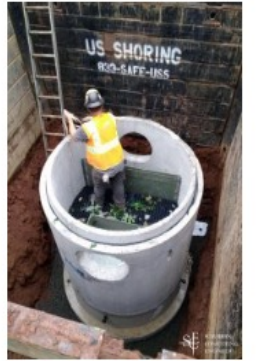
Installation of catch basins to control the flow of storm water as part of Ridgefield Park Village's long term control plan to address CSO's
